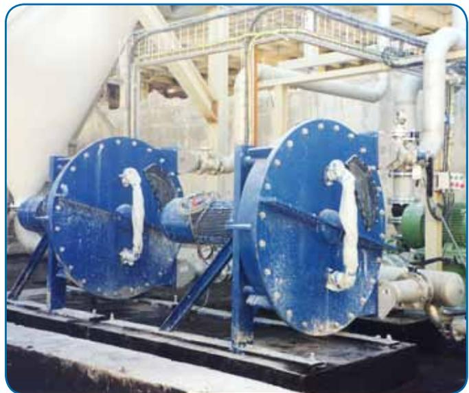
Abaque™ Series Peristaltic (Hose) Pumps possess the operational versatility to reliably handle a wide array of fluids in paint-and-coatings manufacture, from viscous slurries to water-thin liquids.
