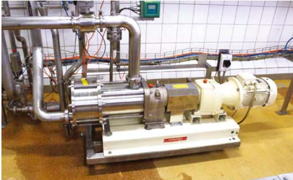
What sets the Mouvex® SLS Series Eccentric Disc Pump apart is an innovative seal-less design that incorporates a hermetic pump head with a self-adjusting eccentric shaft protected by a double-wall stainless-steel bellows that ensure long life and product safety.
