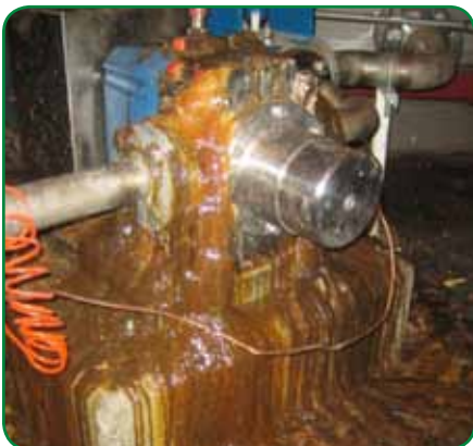
These are a few examples of what can go wrong when pump styles with inadequate product-sealing capabilities are used in resin-handling applications.
