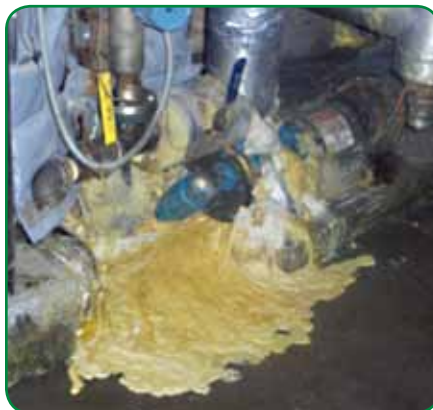
These are a few examples of what can go wrong when pump styles with inadequate product-sealing capabilities are used in resin-handling applications.
