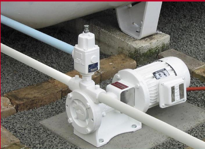
THE EBSRAY MODEL RC SERIES REGENERATIVE TURBINE PUMPS are designed and precision built for high pressure transfer of LPG, Propane, Butane, Autogas, DME etc.
