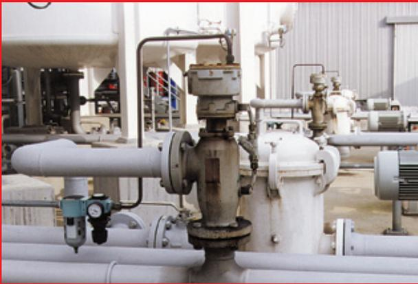
In-Line PFM Systems for modern LOBP operation installed with local control pressure regulator
