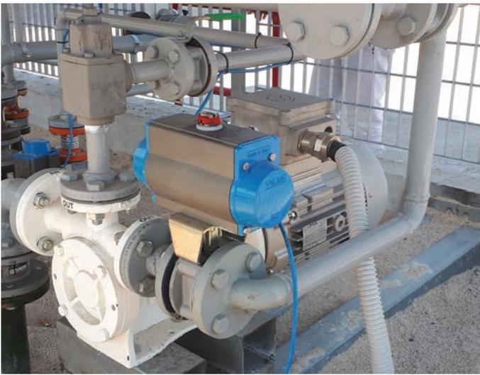
*Regenerative turbine pumps are more energy-efficient because they typically require a smaller motor than competitive technologies, but despite that, they are still able to produce flow rates of up to 160 gpm (600 L/min) or more.*
