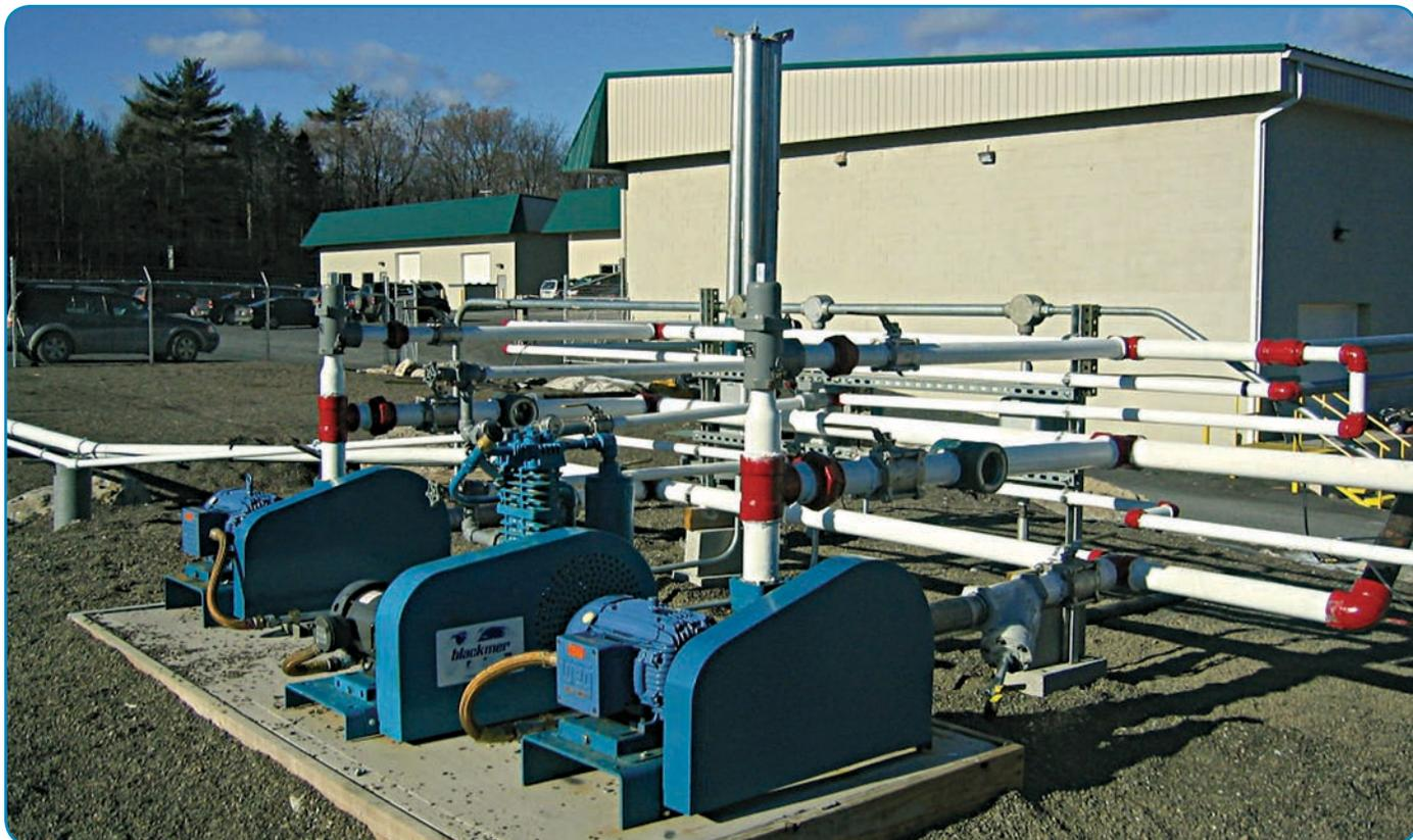
Blackmer LB161 Series Reciprocating Gas Compressors installed at Kingston Oil Supply Corporation's Saugerties, NY, facility for propane gas vapor recovery. The system was installed by Duck Harbor Energy Consultants, LLC, Equinink, PA.
