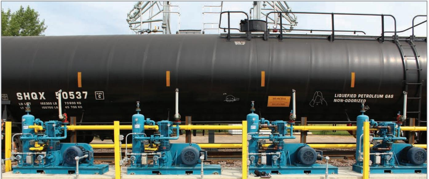
A critical piece of equipment in the propane-railcar unloading process are the compressors that are used to remove the propane from the tankers and transfer it into the storage tanks. To optimize this process, Alliance Midstream utilizes LB942 Series Reciprocating Gas Compressors from Blackmer®.
