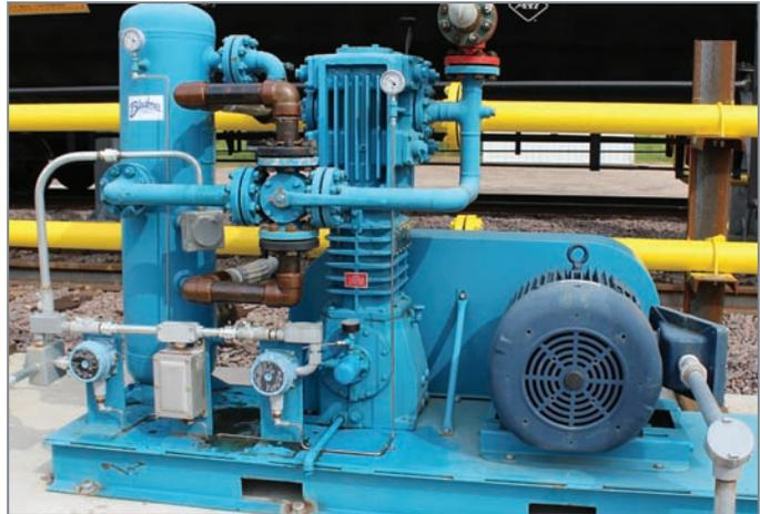
The Blackmer® compressors are ideal for the Alliance terminal's needs because they feature single-stage, oil-free operation and have been designed specifically for propane transfer and vapor recovery.
