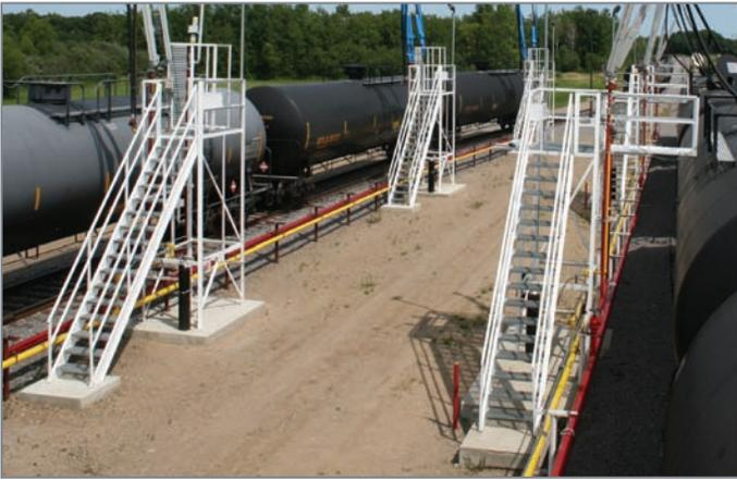
The expanded Rockville Propane Terminal features 10 rail-loading towers and 16 propane-storage tanks with a combined storage capacity of 620,000 gallons. A second loading island was also built, doubling the number of transports that could be loaded in any given day.
