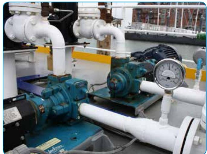
Harbor Fuel 1 is outfitted with Blackmer GX & X Series pumps, a 2-1/2-inch model for high-capacity fuel transfer, and a 2-inch version for operations that require lower flow rates.
