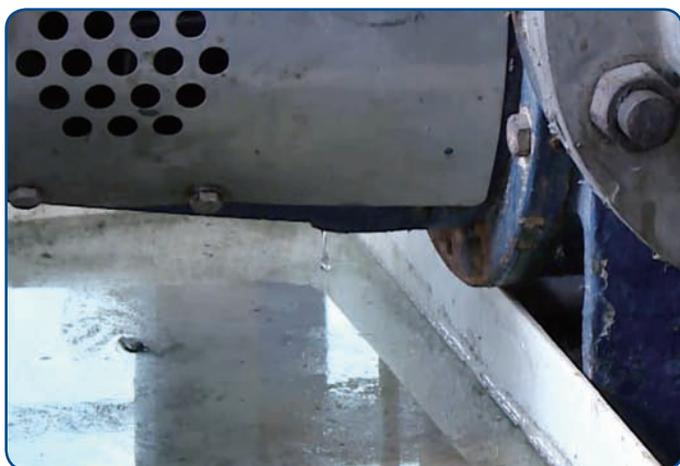
The shortcomings of gear pumps were very serious during production, as leakage would occur every one to two months.
