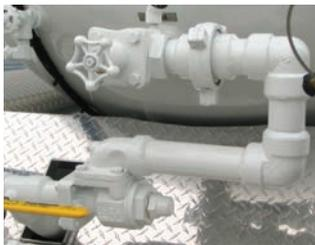
Blackmer differential bypass valves are designed to protect pumps and system components from excessive pressure damage, and no LP gas pump installation is complete without one. Blackmer offers five different models that provide
