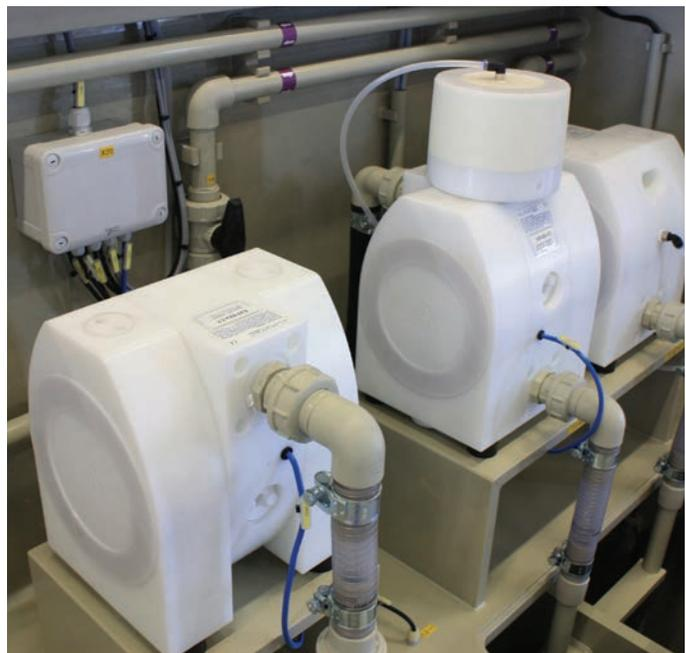
*The design of E-Series AODD Pumps features an optimized flow pattern that allows them to offer increased pumping capacity while consuming less air, resulting in a more cost-effective pump.*
