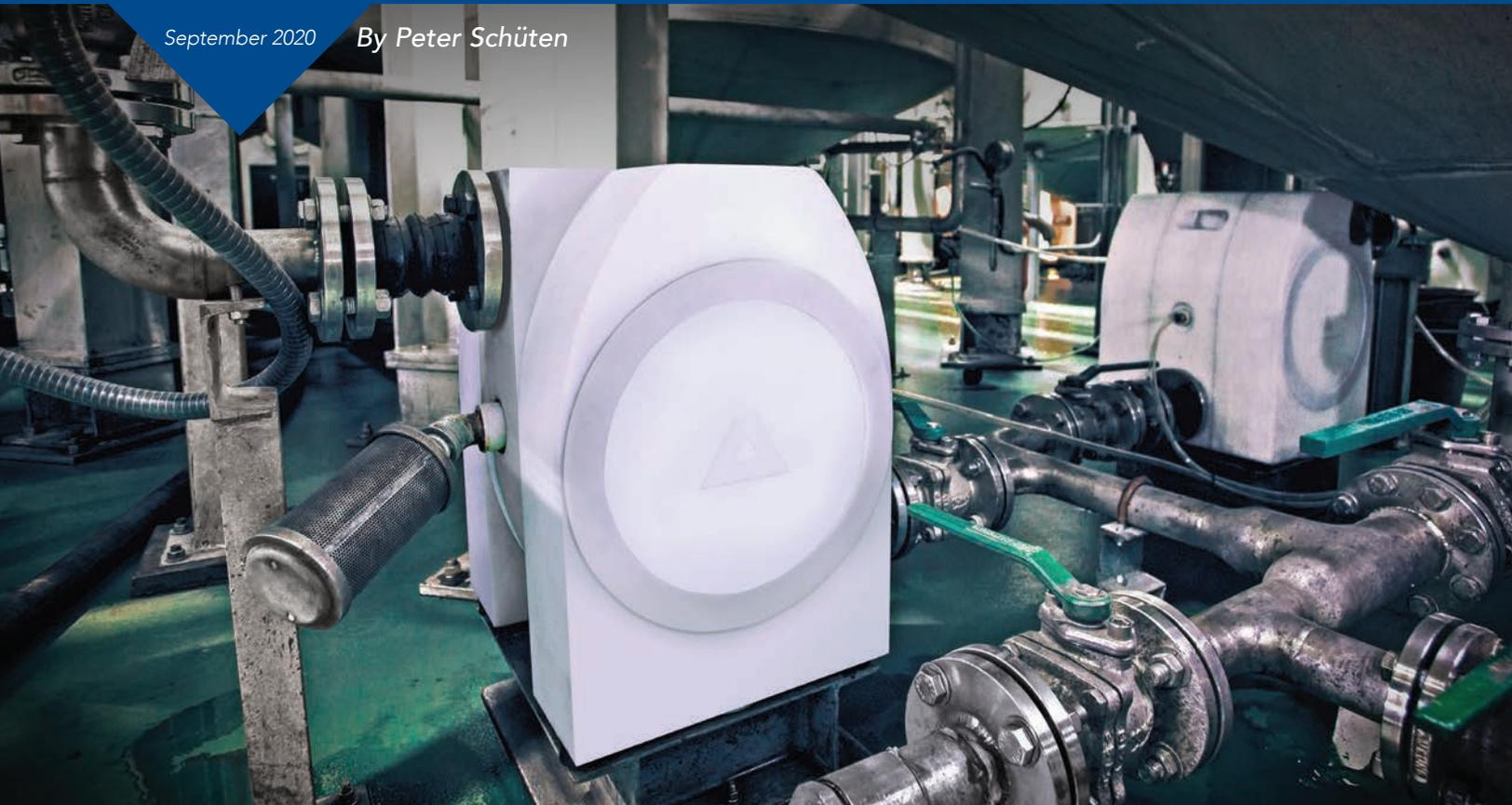
*Almatec® Air-Operated Double-Diaphragm (AODD) Pumps have built a well-deserved reputation as a go-to pumping technology for rugged in-the-field applications that require the safe and efficient transfer of everything from solid-laden slurries to corrosive, abrasive and even explosive materials.*
