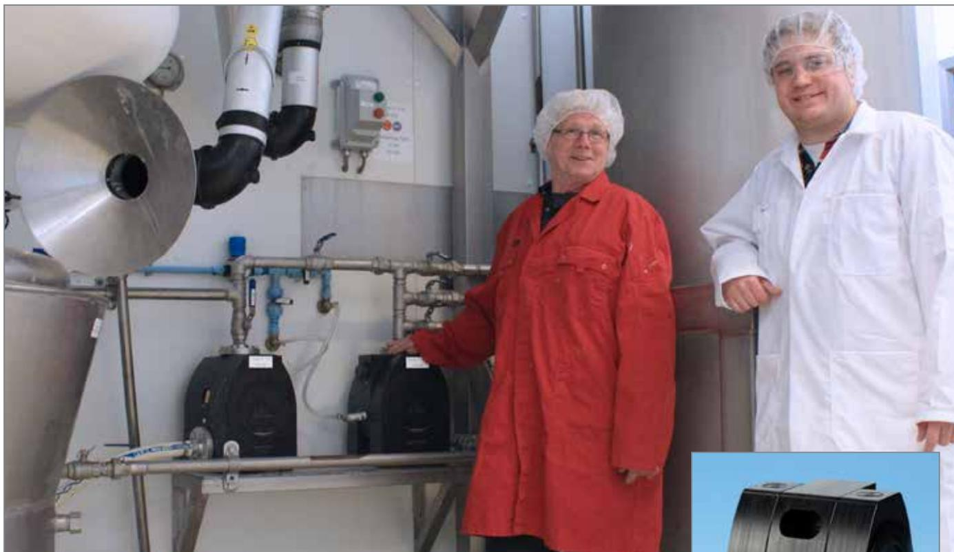
Remco Vree Egberts, right, R&D Manager and Project Leader, and Wim Ekkelkamp, Technical Manager, at Ofichem Group B.V.'s Lab Ofichem API-manufacturing facility have chosen the Almatec® E-Series Air-Operated Double-Diaphragm (AODD) Pump (inset) because of its ATEX certification for handling dangerous materials and leak-free operation.
