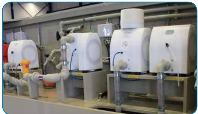
The solid-body, plastic construction of Almatec® E-Series AODD Pumps make them ideal for handling the aggressive and corrosive fluids that are used during the hot-dip galvanizing process for steel, including flux fluid and hydrochloric acid.
